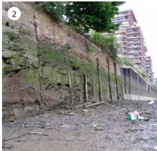
(1) Tidal defences prior to works © Unicomarine copyright and database rights 2013; (2) Tidal defences prior to works © Unicomarine copyright and database rights 2013; (3) Artists impression of the completed tidal terraces © Capita Lovejoy copyright and database rights 2013
